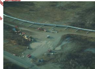
Aerial photo of the Trans-Alaska Pipeline System where the line is supported by rails on which it can move freely in the event of fault offset. Here the line has moved toward the west end of the rails.
