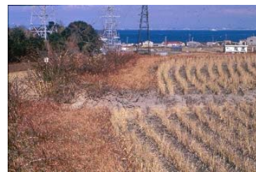
Fault offset in the 1995 Kobe earthquake moved the edge of this rice paddy 6 feet along the fault.
